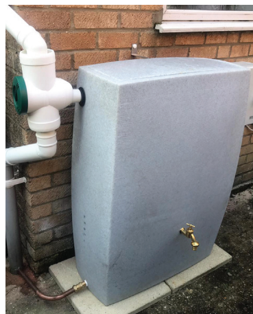
L to R: Nat Flatman Street property frontages and example rear garden smart tank installations.
